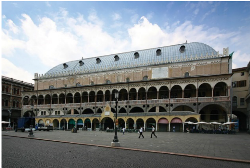
Figura 7: Palazzo della Regione. (Padua,1218). Fuente: fotografía de Stefan Bauer para The Plan Journey, 2009. http://www.theplanjournal.com/article/planning-criticism-operative-contingencies-project-italian-tendenza-0/
