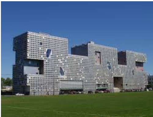
Figura 4: Simmons Hall (Estados Unidos, 1999) Fuente: Benjamin Blankenbelder, "Simmons Hall MIT" 2015. http://www.architecturerevived.com/simmons-hall-mit-massachusetts/
