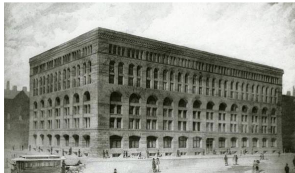
Figura 4. Edificio Marshall Field Wholesale Store. Arq. Henry Hobson Richardson – 1885.
