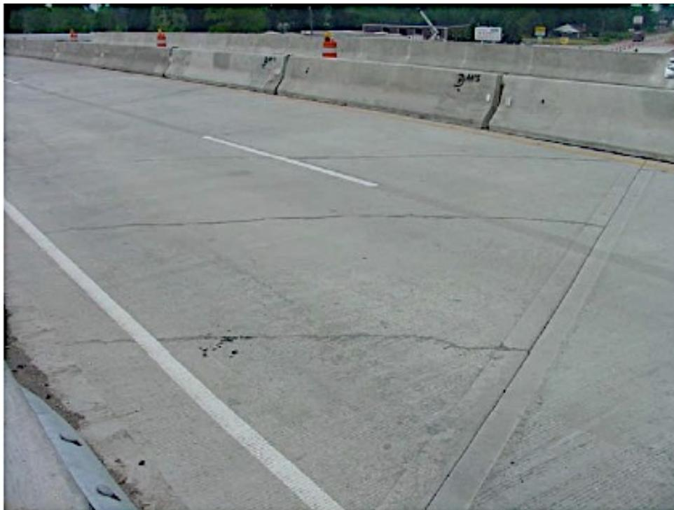
Fuente: GONGKANG FU, Jihang Feng. *Bridge Deck Corner Cracking on Skewed Structures*. 2007. p.8.
