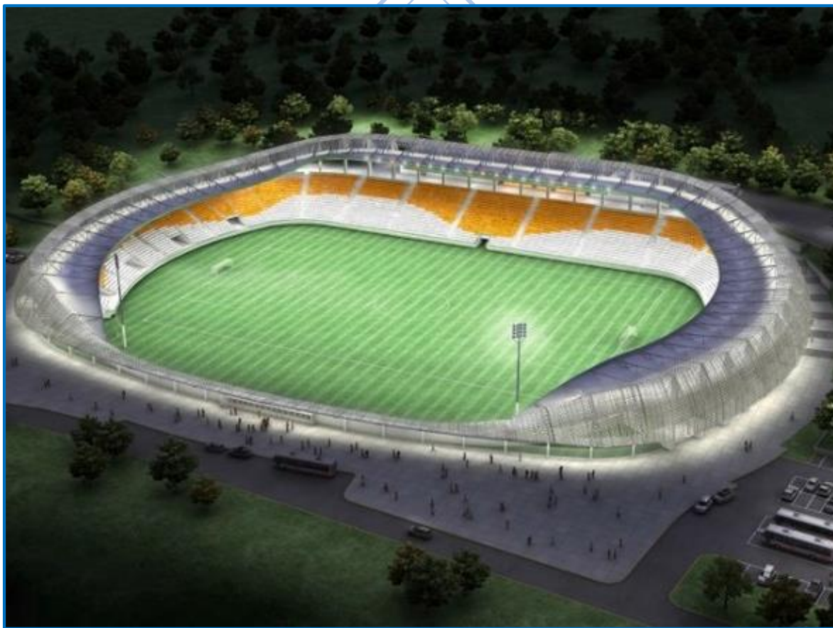
Figura 35 Vista general nocturna
