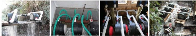
PowerSpout PLT turbines are often installed in multiples to handle higher flows.
