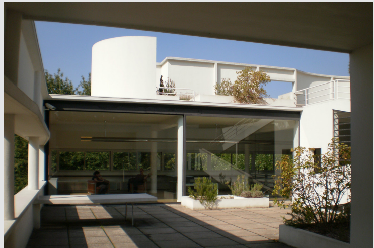
ROOFTOP, VILLA SAVOYE.
