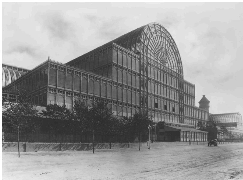
Figura No. 12. Crystal Palace building, London, United Kingdom
