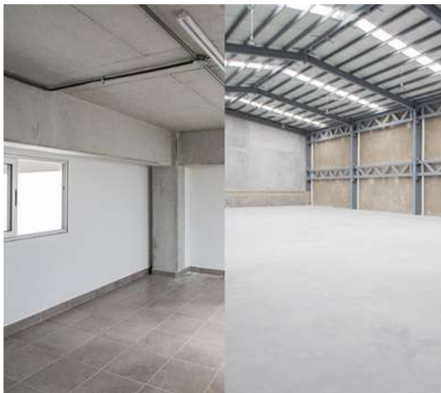
Figura 41, Interior de Ofibodegas, https://assets.vbt.io/public/files/2399/DISTRIBODEGAS_5.pdf
