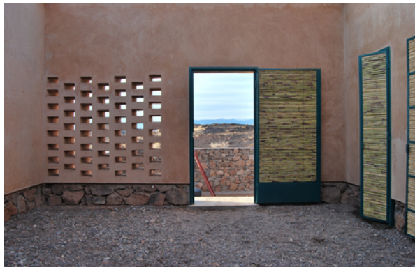
Figura 09. Recinto preescolar Aknaibich / BC architects + MAMOTH. 2014
