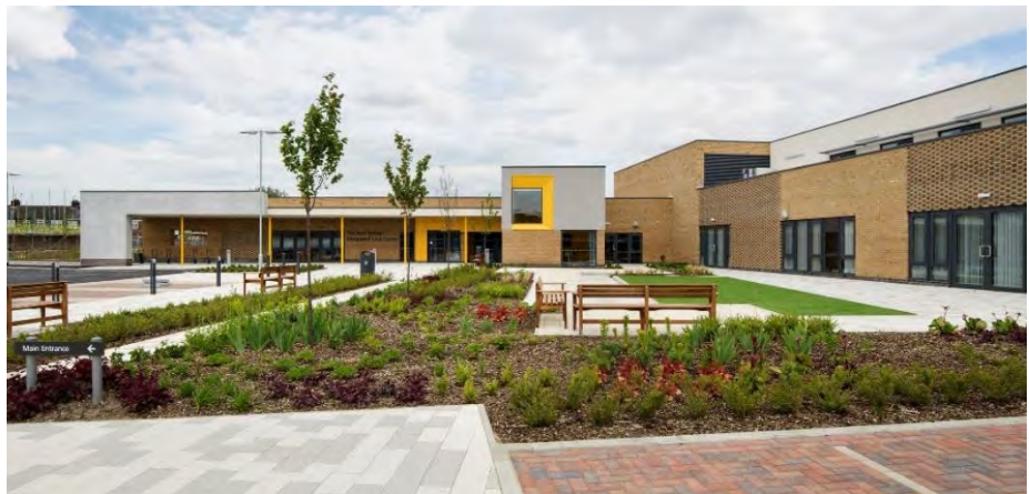
IMAGEN 8. Exterior del Centro de Atención Integrada, Jean Bishop. Fuente: https://archello.com/project/the-jean-bishop-integrated-care-centre Autor: Jill Tate
