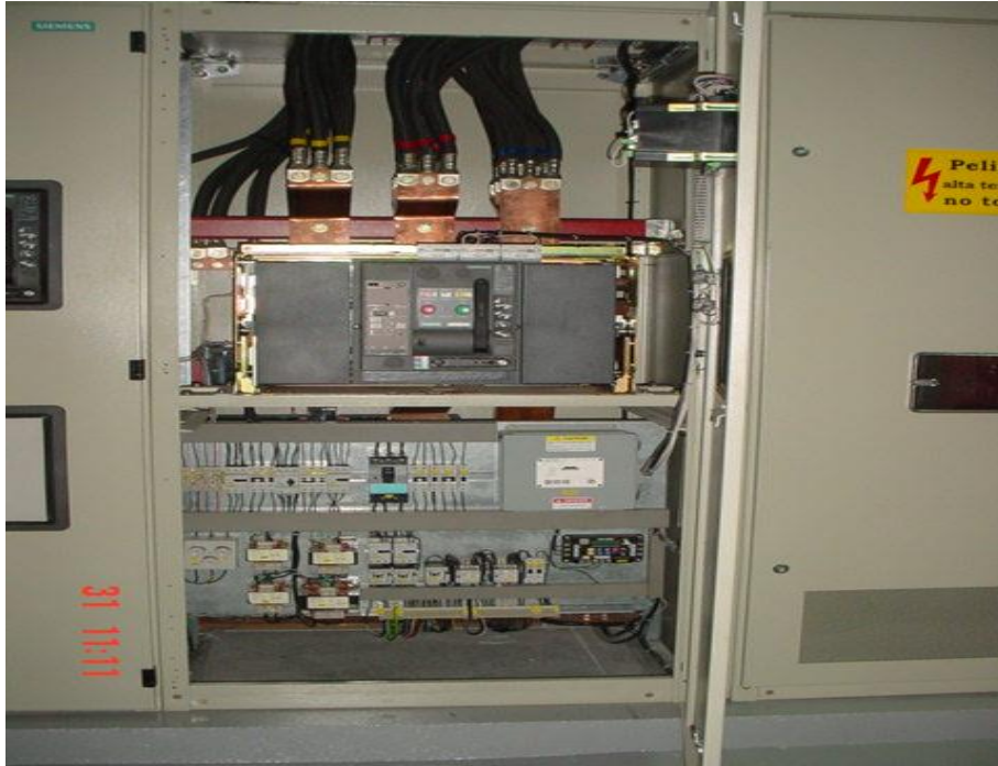
Figura 7. Interruptor principal WL III 5 000 H
